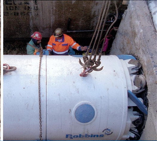
LEFT: The Robbins 72-inch (1.8 m) Motorized SBU (SBU-M) broke through almost exactly on line and grade after 395 ft (120 m) of boring. RIGHT: The Robbins SBU-M was the largest machine of its kind ever made, and utilized a mixed ground cutterhead in clays as well as rock.
